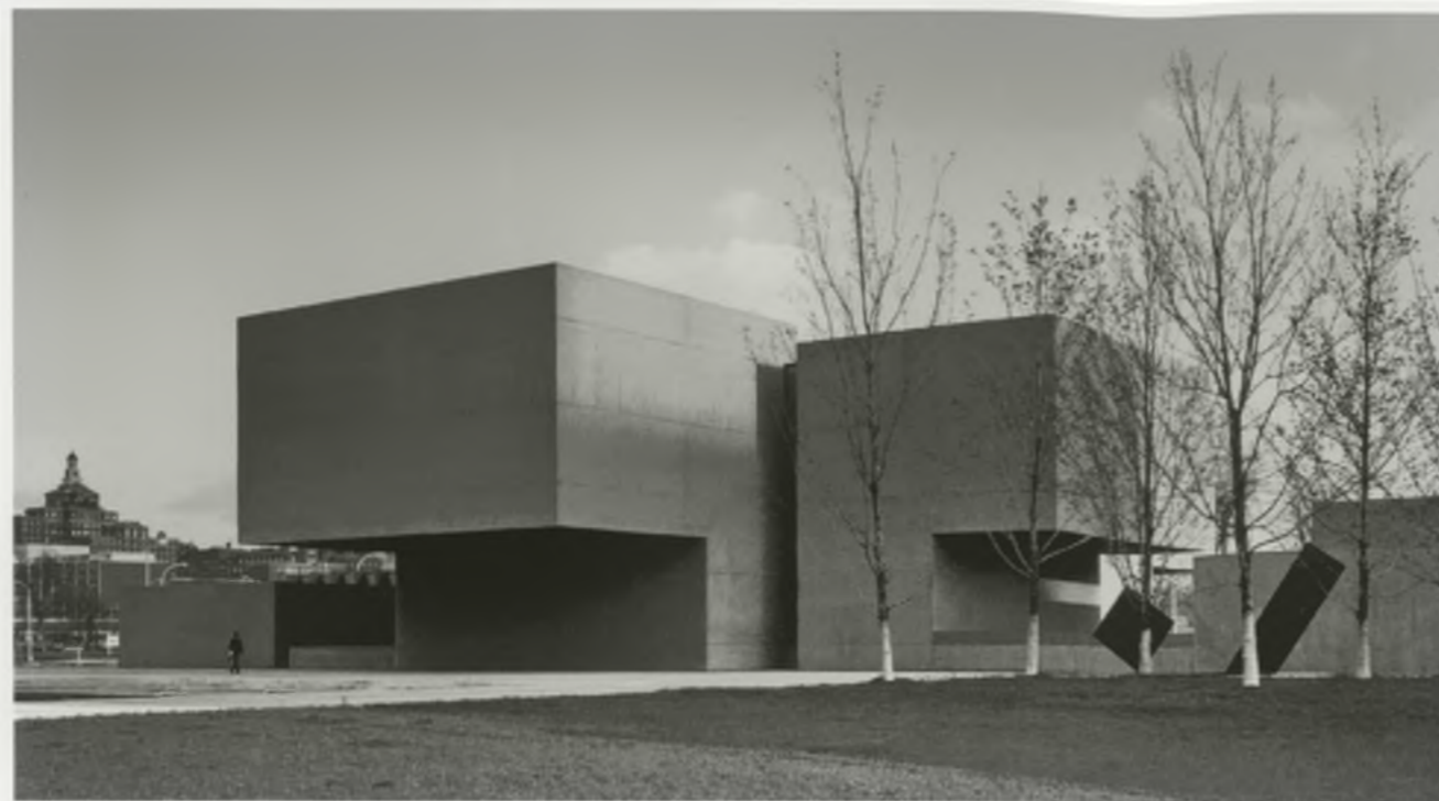
4. Edward Larrabee Barnes, Walker Art Center, Minneapolis, 1966–1971 Walker Art Center, Minneapolis
